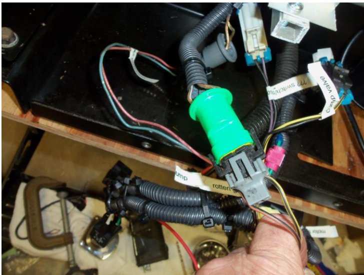
The switch housing from the RGS. It connects with its matching factory connector because the factory wiring harness was not altered.
