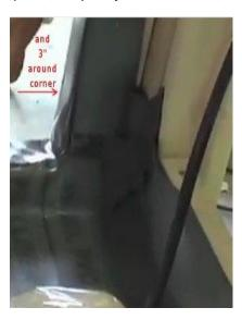
• The liner is seldom run beyond the front of the threshold/curb/dam as required by the code. The FBC-Residential requires that the shower liner be extended a minimum of 3" beyond the dam, and a minimum of 3" around the corner and face of the wall if the wall is that configuration – see configuration in above photo.
